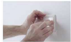
04 Mount the cover of the pushbutton.
