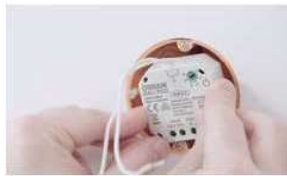
02 Place the DALI PCU into the flush box.
